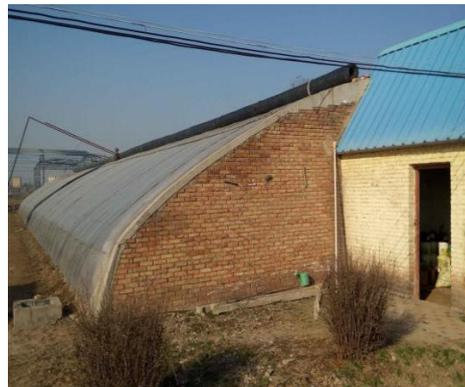
Figure 1. Solar greenhouse in China
